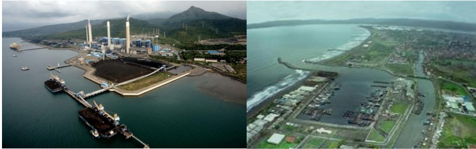
Paiton Power Plant Coal Port
